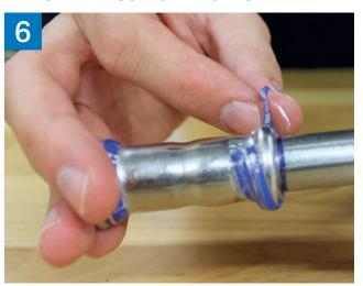
Remove pressing indicator. Check the correct insertion depth has been met.
