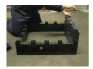
Invert the assembled section & put a full collar (40cm deep) on all the bosses Fit one side panel, then an end panel, then another side panel & finally another end panel
