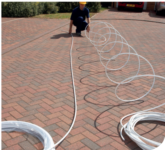
Figure 4: Hep 2 O pipe (left) comes off the coil straight
