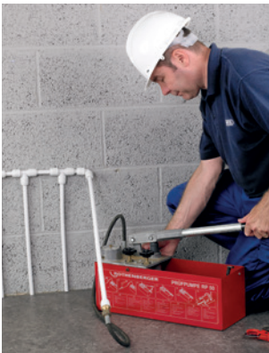
Figure 59: Pressure testing
