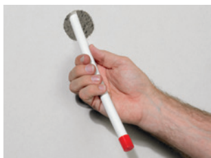
Figure 22: Always protect pipe ends
