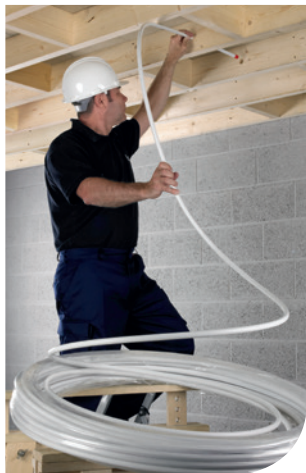
Figure 23: Packaging retains pipe until last metre
