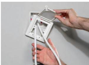
Figure 52: Installation procedure of HX113 cover plate
