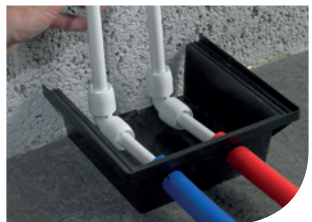
Figure 40: Cut conduit box for wall termination
