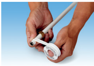
Apply PTFE tape if required
